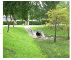
**Grassed swales** can be found directing storm water around buildings and towards the pond. Inlets are found in parking areas, depressed green spaces, and curbs, and are usually underground conveyances directing the runoff into the pond.
