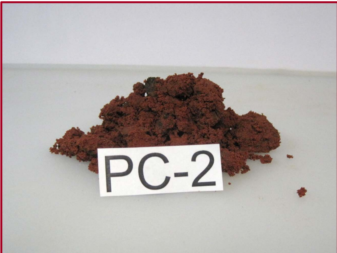
FIGURE 5D: PHOTOGRAPH OF SAND-CLAY BASE (LBR 75) ENCOUNTERED AT PAVEMENT CORE PC-2
