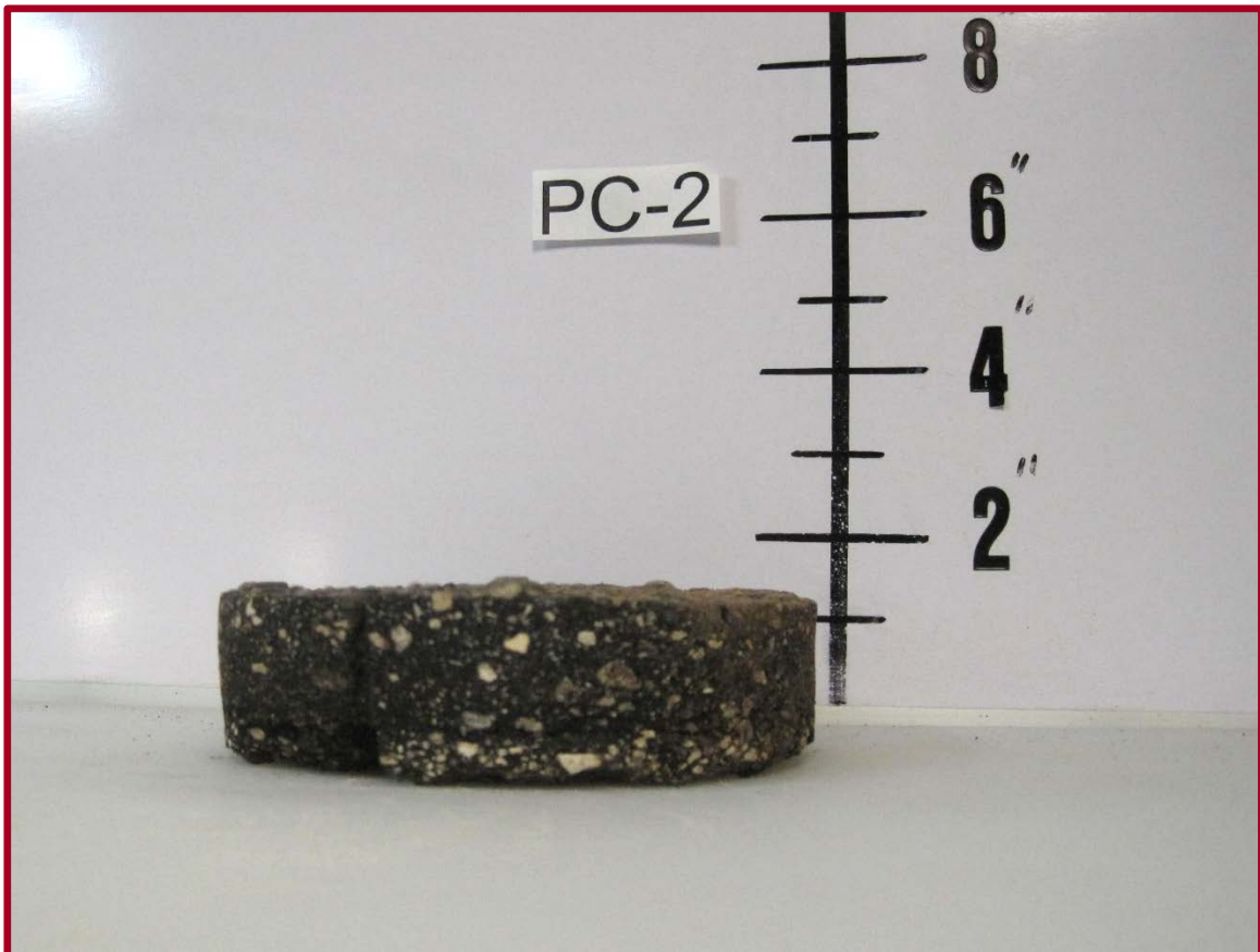
FIGURE 5B: PHOTOGRAPH OF PAVEMENT CORE PC-2 (NOTE: PHOTOGRAPH DOES NOT DEPICT FULL DEPTH OF ASPHALT STRUCTURE)
